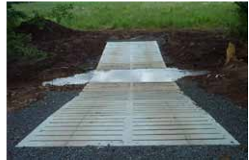
A cattle crossing like this one helps stop erosion by preventing cows from trampling streambanks.
